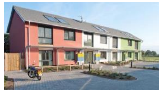
Wimbish Passivhaus certified. (© Hastoe Housing Association).
