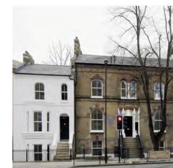
Akerman Road, London (Source: 15-40 Architecture)
