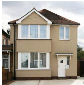
Grove Road, London (Source: Bere Architects)
