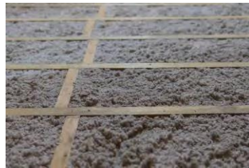
Cellulose- made from recycled paper (Source: Eco Spray Insulation)
