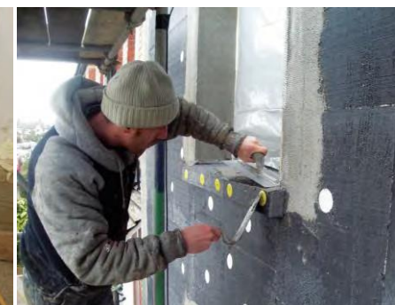
Window install in EnerPHit retrofit (Source: Passivhouseplus)
